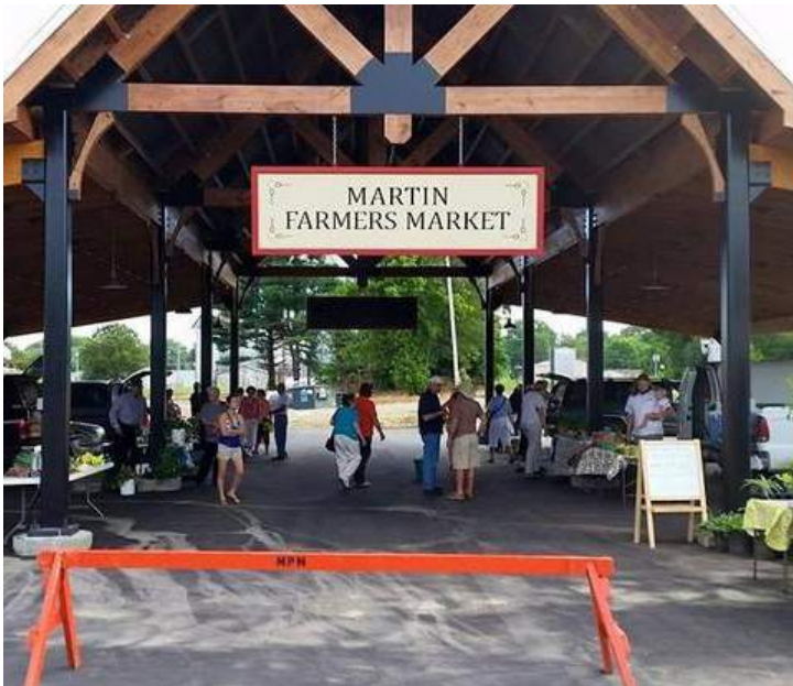
Both of the examples on the bottom of this page are good examples of how to execute the pavilions. This image features traditional heavy timber construction with painted metal plates.
