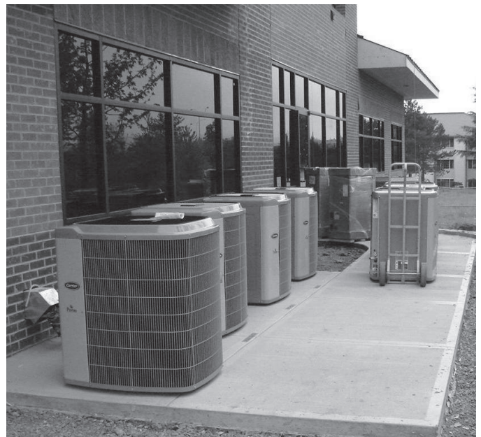
HVAC equipment without screening must not be permitted. Screen walls, architectural enclosures, fences, and landscaping must conceal these elements from public view.
