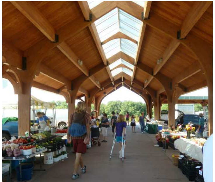
Pre-engineered glue laminated wood members provide the warmth of traditional wood framing, but the structures are much simpler in design.
